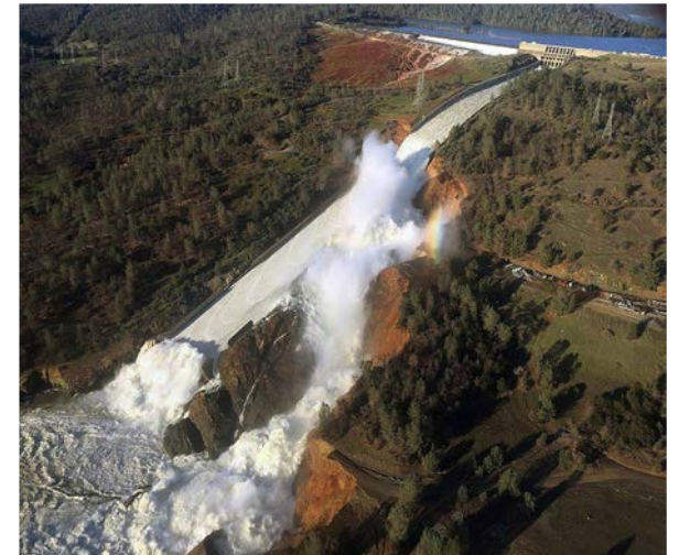
Damaged spillway at Lake Oroville in Feb. 2017
