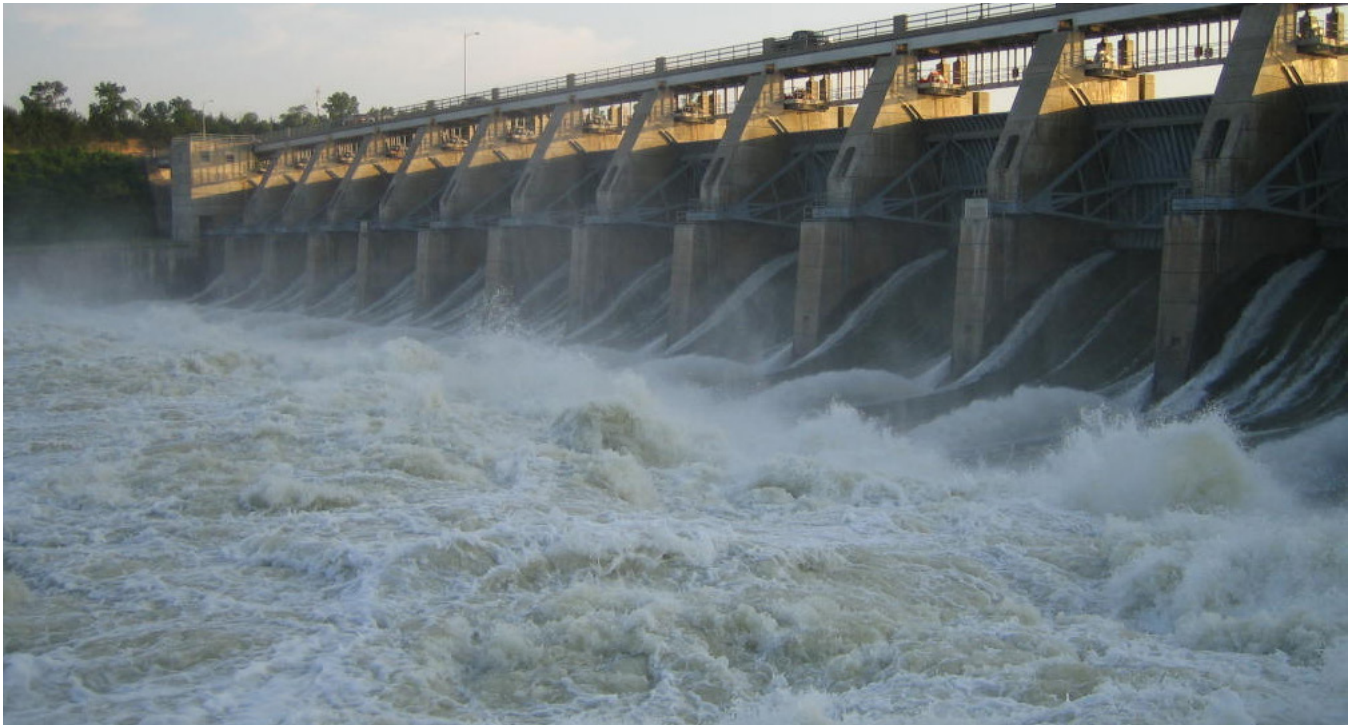
Gavins Point Dam is located on the Missouri River in Nebraska and South Dakota
